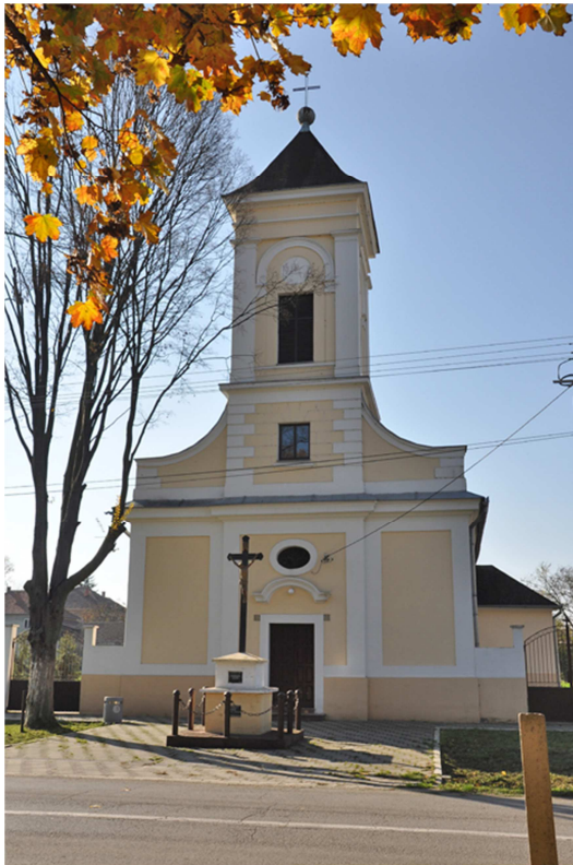
Figure 5. Catholic church in Opovo from 1776 (October 2022, image: Z. Cvetkovic)
