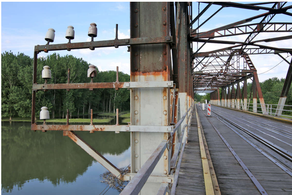
Figure 6. Bridge across the river Tamiš on the railway Zrenjanin - Sečanj
