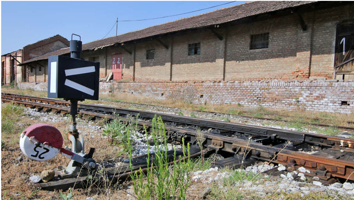
Figure 20. Warehouse in the Vršac station
