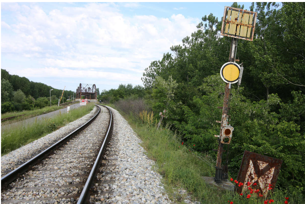
Figure 19. Mechanical traffic lights at the Orlovat - Tomaševac railway. These were used to control traffic on the bridge over the Tamiš River.
