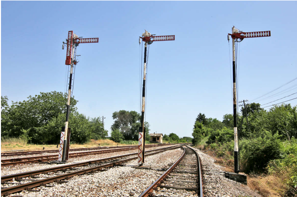
Figure 17. Mechanical traffic lights at the Alibunar station
