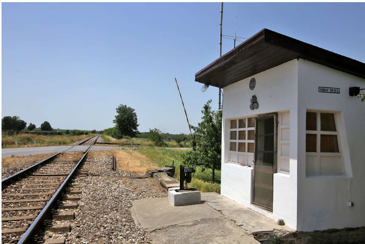
Figure 14. Guard house in Alibunar at the entrance of the station and nearby the level crossing. At the front of the guard house, there are switches for controlling the road ramp.
