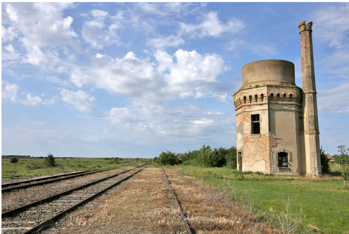
Figure 11. Water tower in Orlovat
