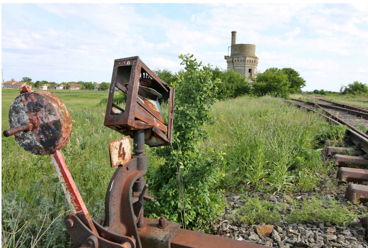
Figure 15. Operating switch in Orlovat. It is made in 1916 in Graz.
