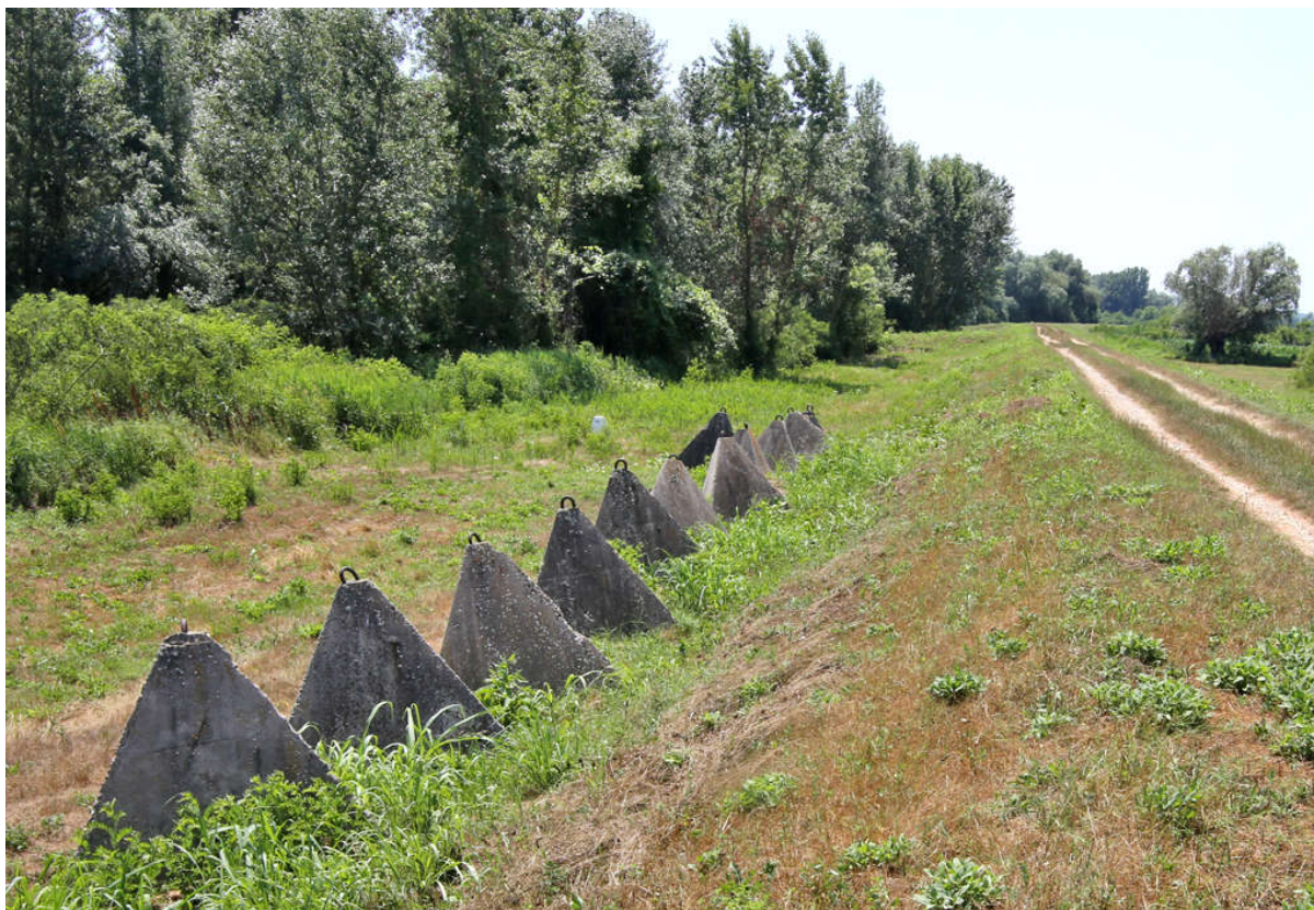
Figure 3. The railway embankment in the border area alongside the Nera River and old anti-tank barriers.
